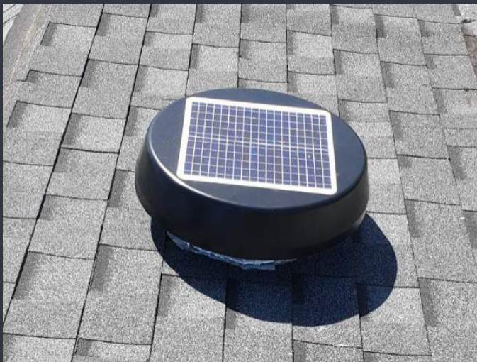
Solar roof ventilation fan reduces internal temperature and provides better air circulation
